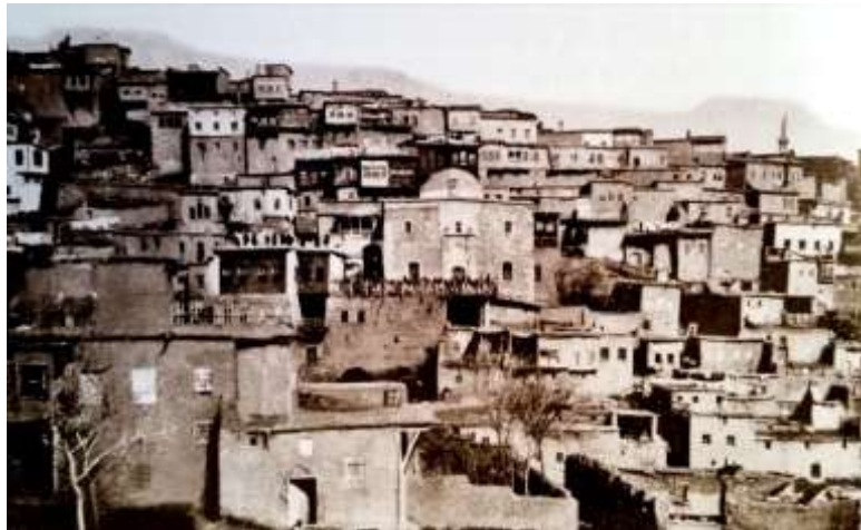
Figure 11. Surp Hagop Church (Source: Veli Sevin-Necla Arslan Sevin-Haydar Kalsen, Ottoman Life in the Castle Neighbourhood of Harput, p. 70)
