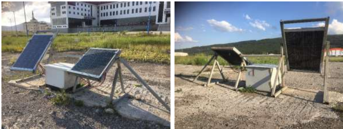
Figure 2. Solar panels are installed on south-facing
