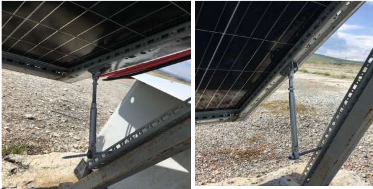
Figure 3. Adjustable screw is used to adjust the tilt angle of the panels
